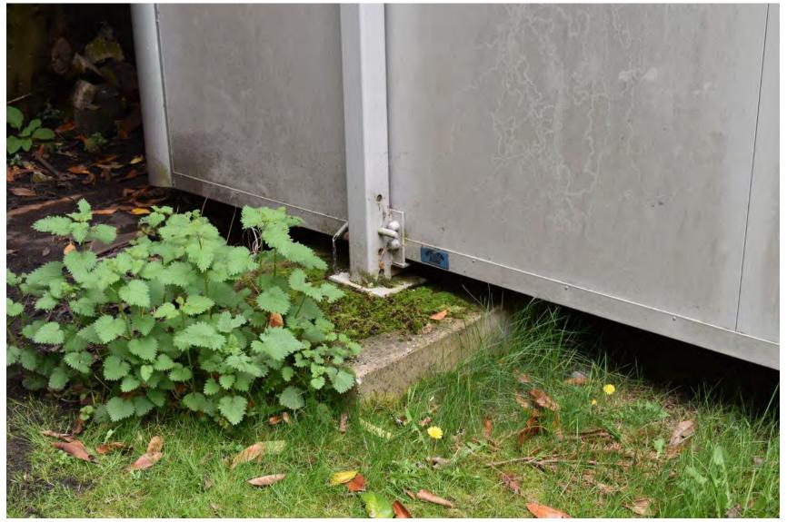
Plate 12: One of the existing Portakabins concrete pads
